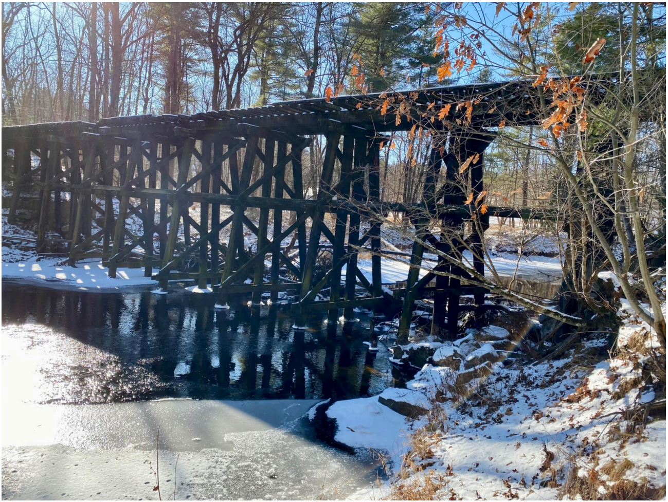
Figure 5. Trestle 2 in West Townsend
