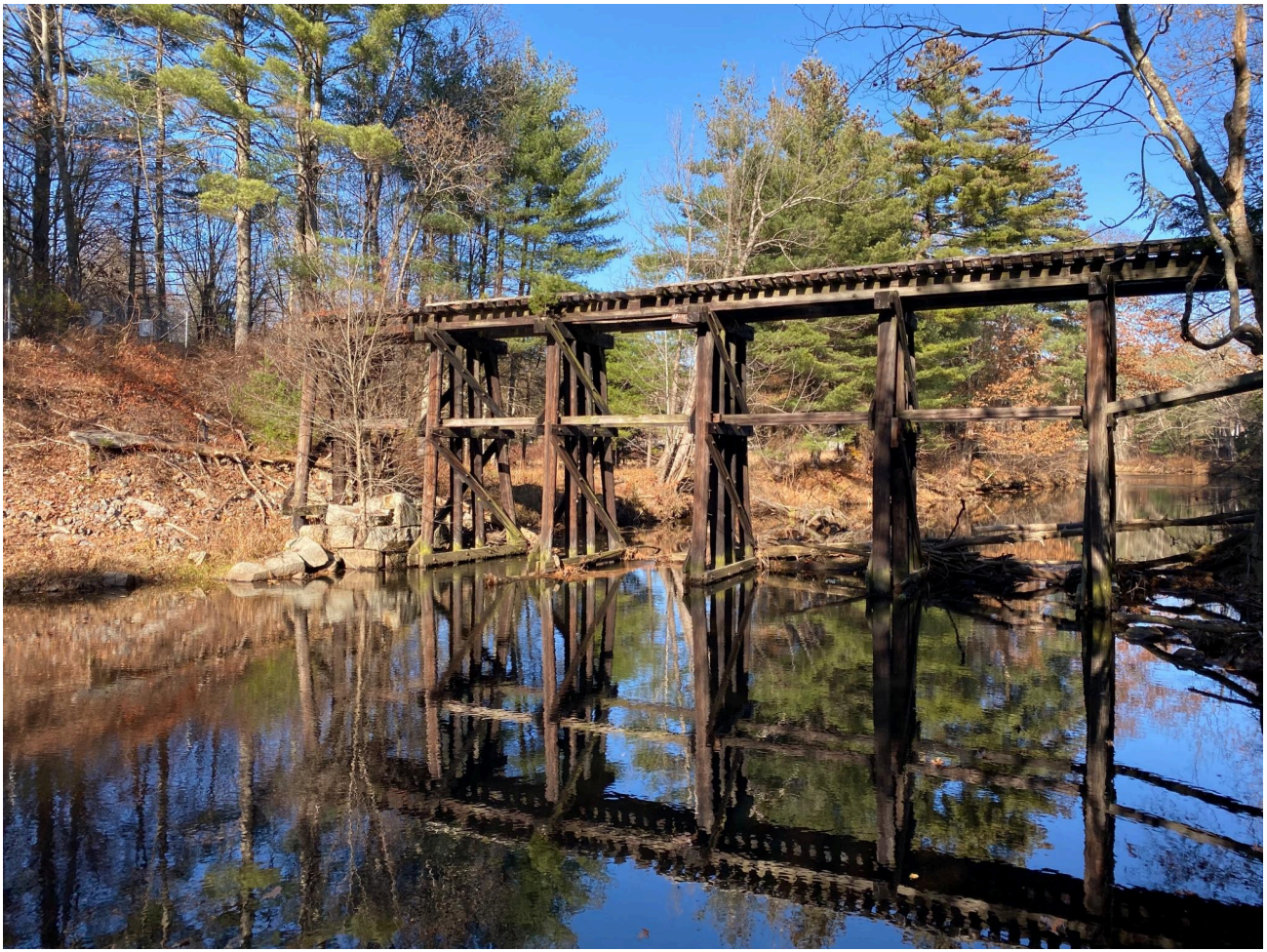
Figure 4: Trestle 1 (near Townsend center)
